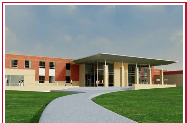
In its 110,000-square-feet of new space, the remodeled Butler High School will contain many new classrooms, including science, music, business, computer, and special education rooms, a wood shop, media center, dining facilities, and administrative offices.
